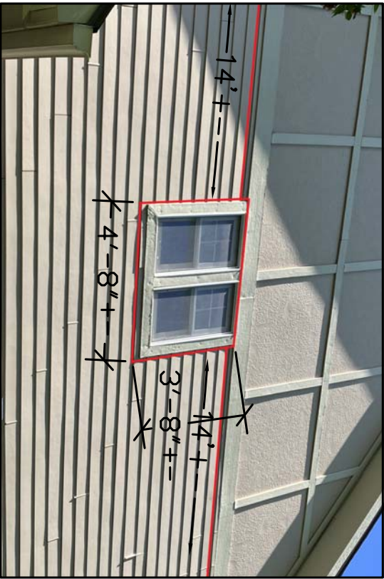
13 7624 JASMINE— SOUTH ELEVATION REPLACE WINDOW TRIM & HALF PIECE OF SIDING WITH FULL PIECE—CAULK & PAINT
