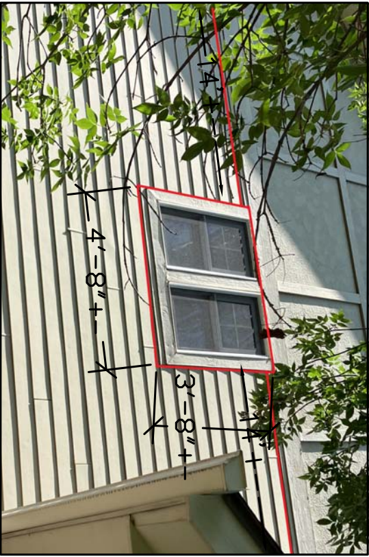
14 7625 JASMINE—SOUTH ELEVATION REPLACE WINDOW TRIM & HALF PIECE OF SIDING WITH FULL PIECE—CAULK & PAINT
