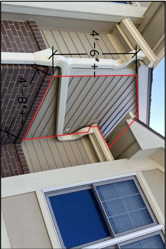
10 7619 DAPHNE – GABLE WALL REPLACE & PAINT DAMAGED SIDING
