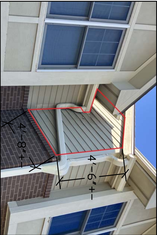
24 7507 WISTERIA – GABLE WALL REMOVE, REPLACE AND PAINT SIDING
