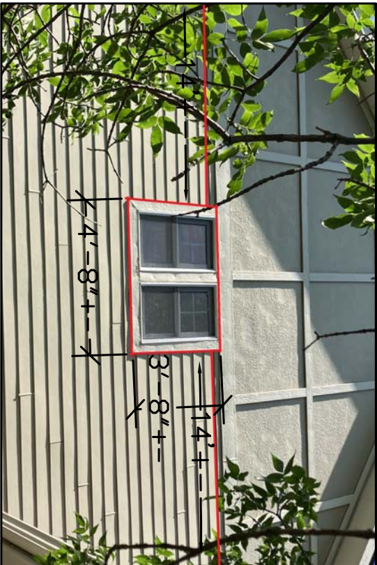
11 7627 DAPHNE – SOUTH ELEVATION REPLACE WINDOW TRIM & HALF PIECE OF SIDING WITH FULL PIECE – CAULK & PAINT
