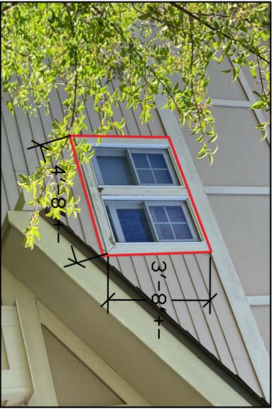
06 7602 DAPHNE-NORTH ELEVATION REPLACE WINDOW TRIM & SMALL PIECE OF SIDING SIDING BELOW-CAULK & PAINT
