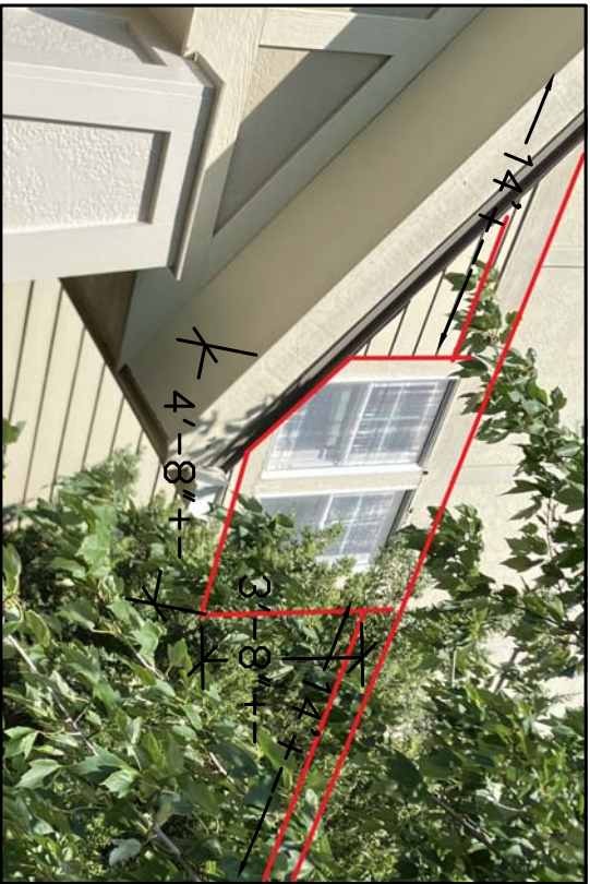
21 7520 WISTERIA – SOUTH ELEVATION REPLACE & PAINT TRIM & SIDING WITH FULL PIECE
