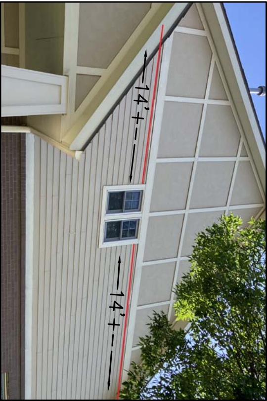
08 7603 DAPHNE-NORTH ELEVATION REPLACE HALF PIECE OF SIDING WITH FULL HEIGHT PIECE-CAULK & PAINT
