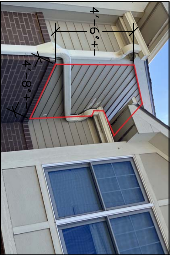
15 7617 JASMINE – GABLE WALL REPLACE & PAINT DAMAGED SIDING
